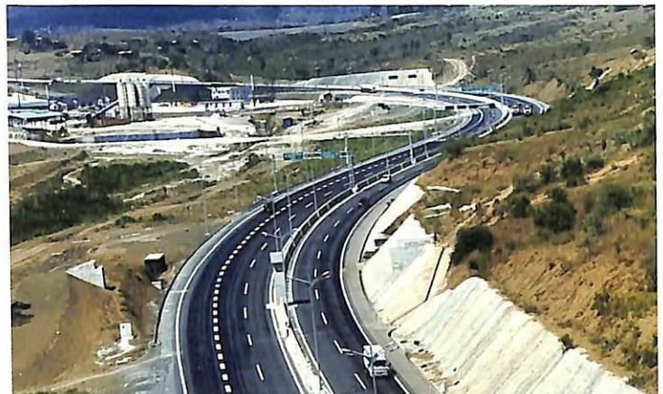
A section Mombasa Port Road Area Development Project.
