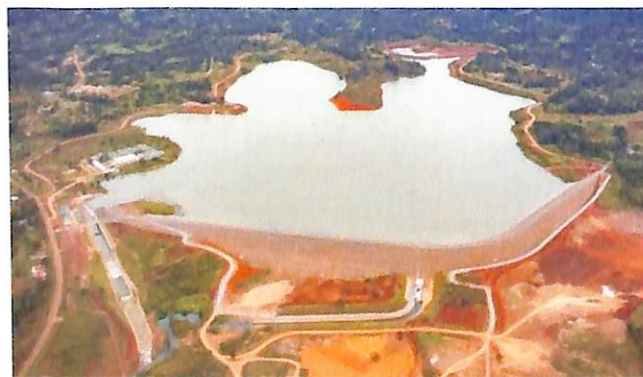
Thiba Dam, completed in 2022 under the Mwea Irrigation Development Project.
